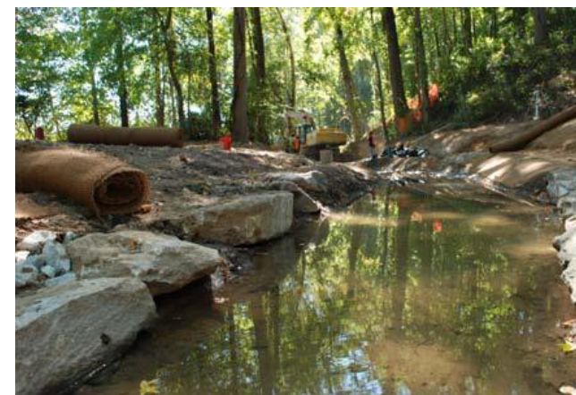
Figure 9-4: Section of East Jesters Creek during restoration – re-establishing connection to floodplain
